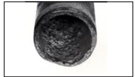
Figure 7-3. Oxygen in the system speeds corrosion (oxidation) of pipes, causing pitting such as shown here.
